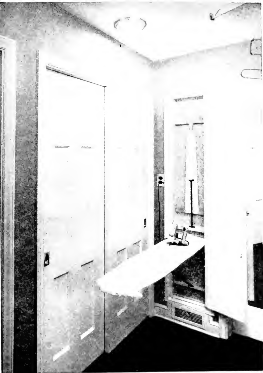
A ceiling fixture above the ironing board casts unshadowed diffused light on the work.
